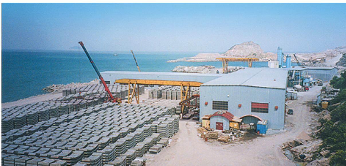
View of Precast Unit at Niu Tou Island, Zhuhai, PRC
