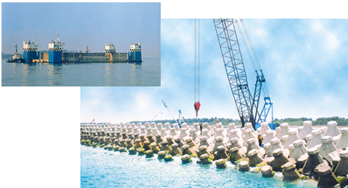
Anping Harbour Outer Breakwater and Lighthouse Works, Taiwan
