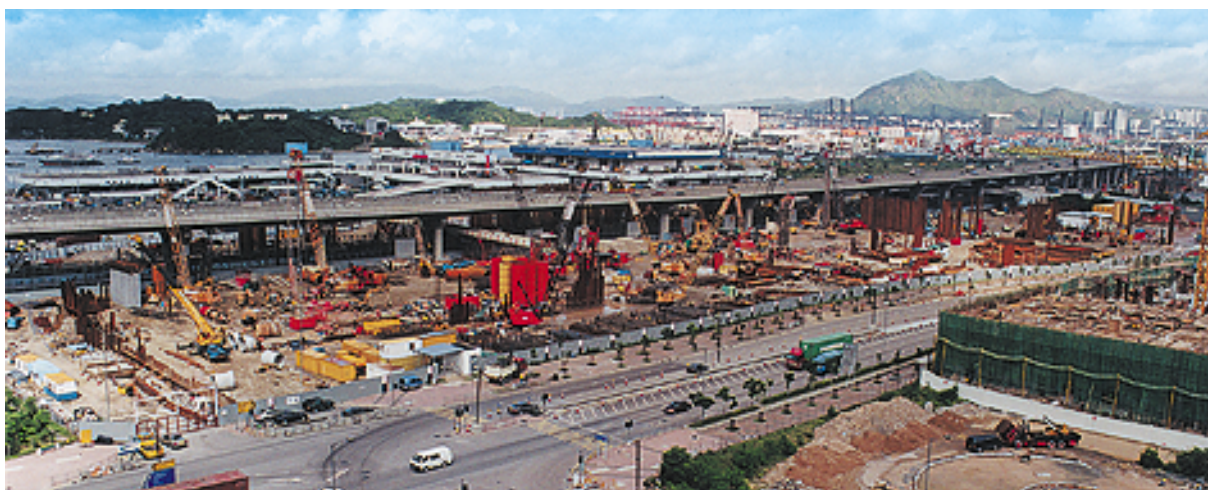
KCRC West Rail Contract CC-402 Nam Cheong Station
